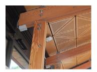
Above: the photograph shows the fixing detail for a roof beam and column - in this instance an integrated flitch beam is secured by stainless through bolts.
