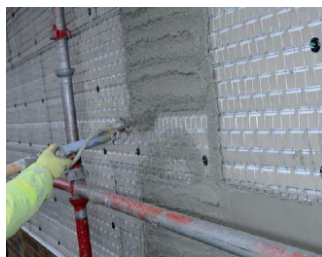
Base Coat Application
